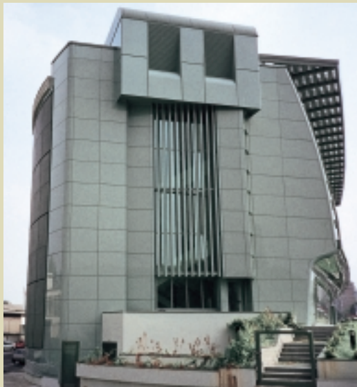
Example of building facade embellished with expanded metal
