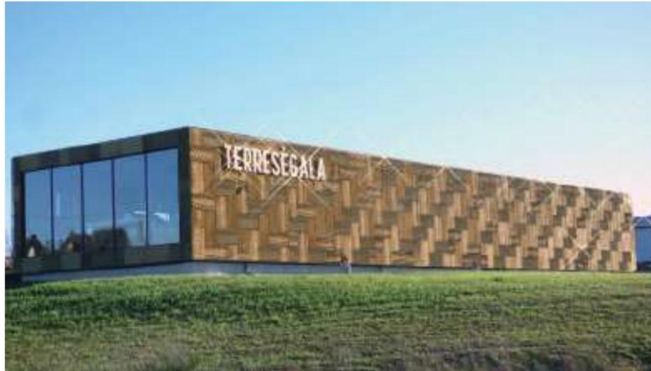
*The panels of this structure were mounted in all four possible positions. In this way the different shades of the golden color are enhanced to obtain a pleasant 3D effect of the façade.*
