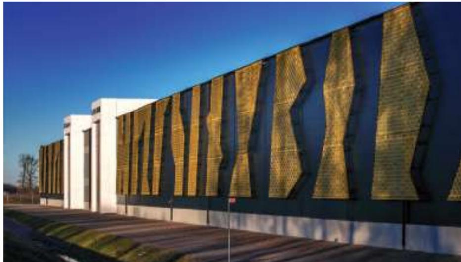
*The structure is composed of 3.200 x 2.000 mm self-supporting panels with welded and shaped profiles in order to form letters in the "runic" alphabet with a height of over 9.5 meters. The design of the substructure includes punctual fixings on a black sandwich panel. The backlight enhances the gold color and the transparency of the expanded metal mesh.*
