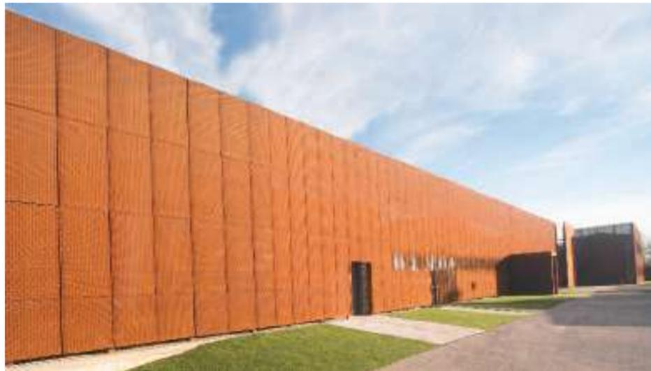
*This renovation project was born to uniform a series of old buildings with a corten masking that would change color over time. In front of the windows, the transparency of the mesh has been increased gradually compared to the parts that covered the wall. This allows the entry of more natural light and a better view in the glazed areas, while it is designed to hide the masonry areas more. The panels are provided with welded profiles and are mounted with a bayonet fitting system.*
