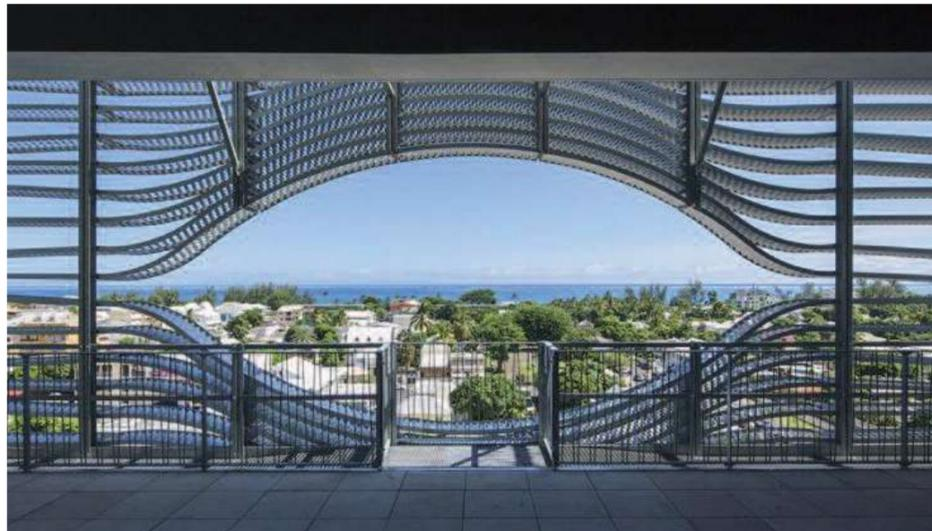
*The library is made by 9.700 pieces, of those 1.200 are unique. The architect wanted to recreate different faces and eyes on the surface. The former was obtained by widening some panels of 400-500 mm, whereas the latter were created with a composition of unique curved pieces.*
