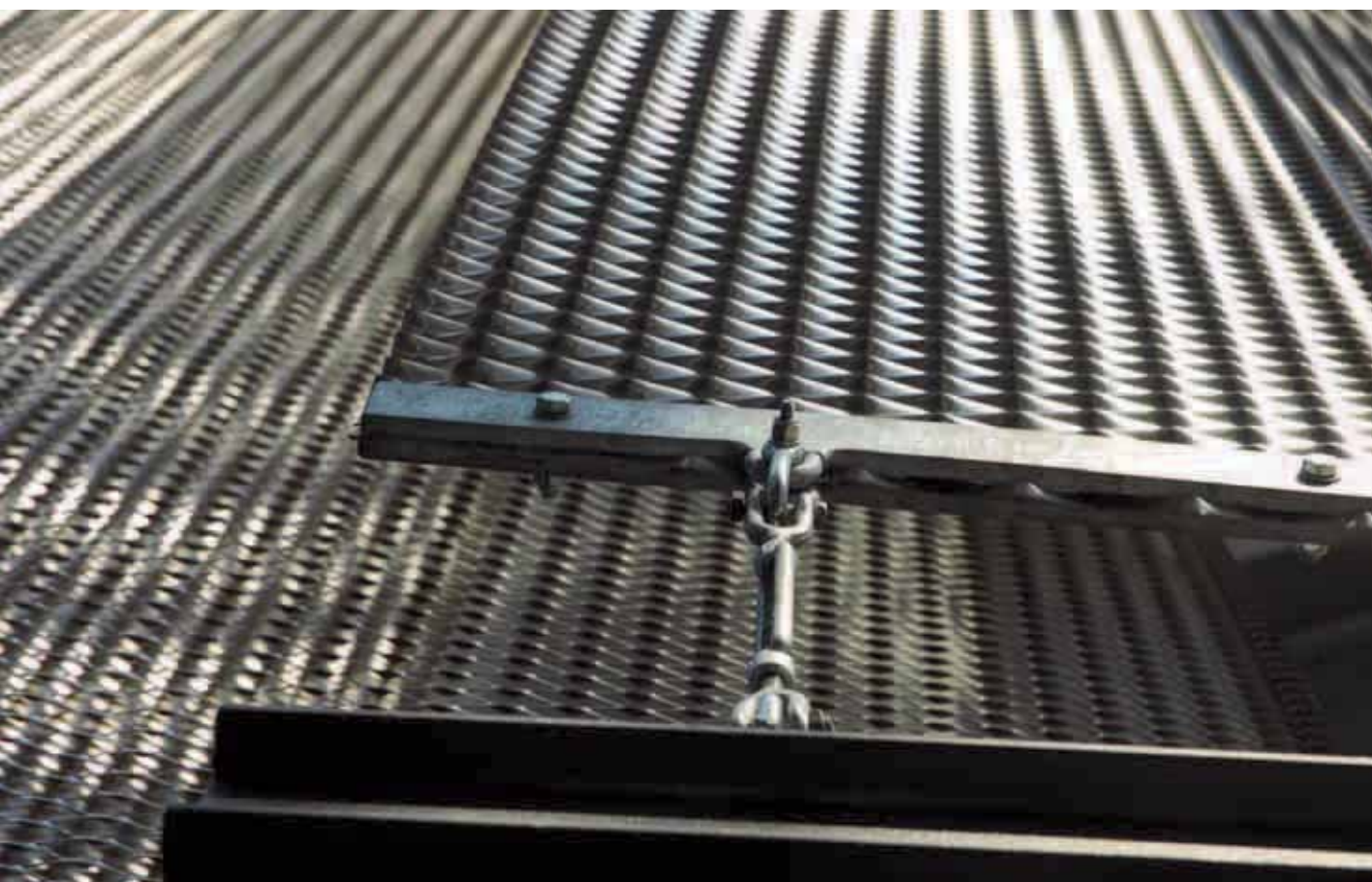
Anchoring of the strip at the bottom.
