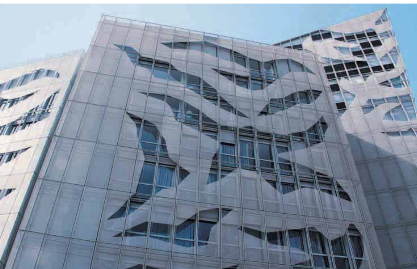
The large façades are decorated with "birds and clouds shaped rips" in the expanded mesh.
