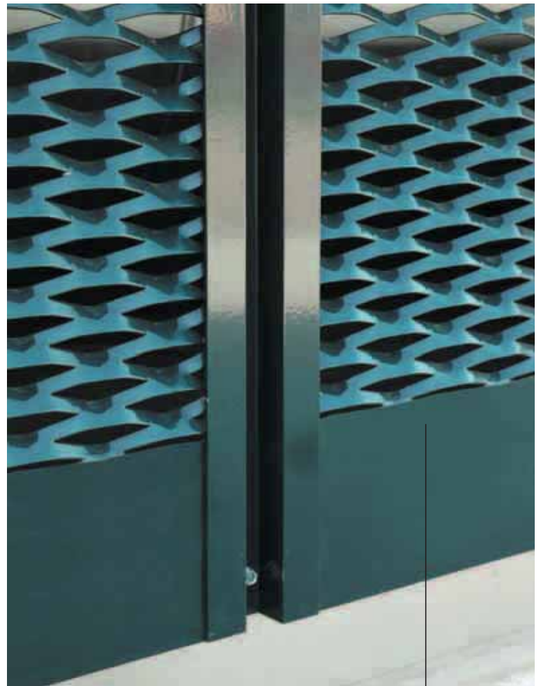
Detail of the junction between the open expanded metal and the solid metal.
